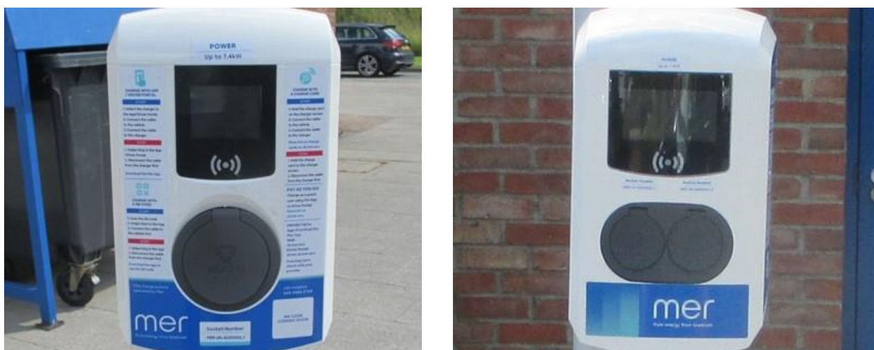
Figure 7: Close-up view of charging devices showing card reader symbol below screen
