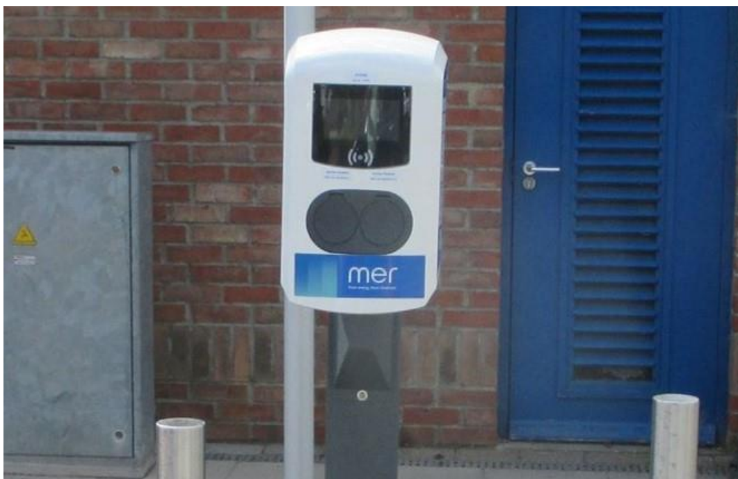
Figure 3: Task 3 Chargepoint with 1065mm socket-height with visible screen reflections
